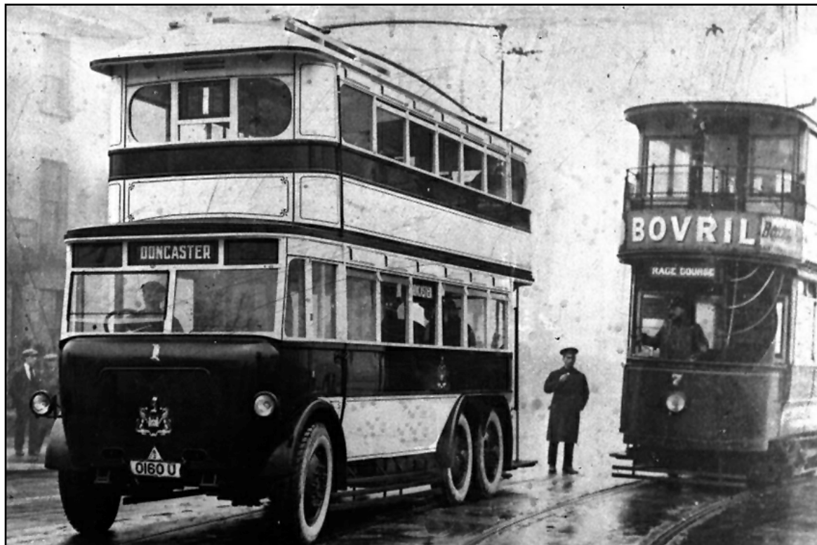
On what looks like a trial run, trolleybus No. 1 (DT821) a 1928 Garrett with Roe H32/28R bodywork is passed by tram No. 7 en route to the racecourse. (LTHL collection).
