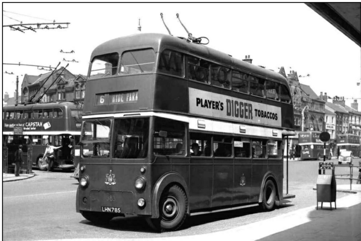
No. 383 (LHN785), seen here in St. Sepulchre Gate in 1958, was an ex-Darlington Corporation BUT9611T chassis with East Lincs 56-seat bodywork new in 1949 and acquired by Doncaster in 1952. (John Kaye).
