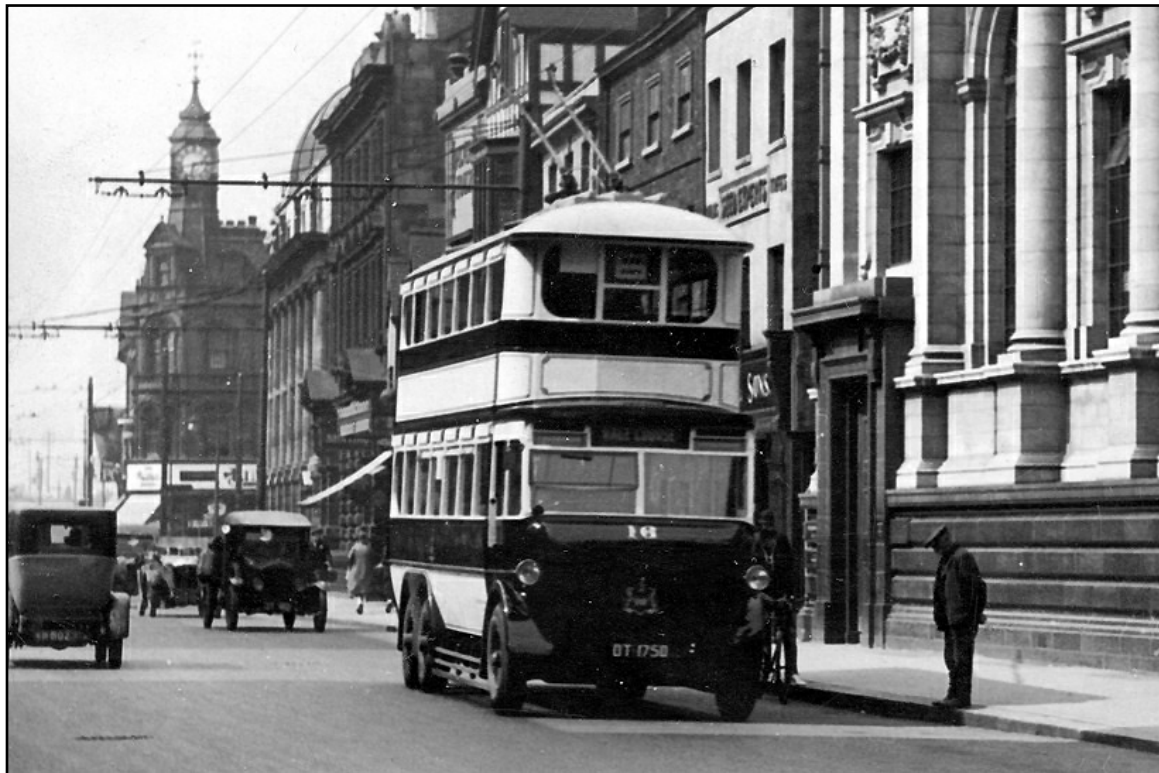
No. 16 (DT1750) was a 1929 Karrier-Clough E6 trolleybus with Roe H32/28R bodywork. It was withdrawn in 1945. (LTHL collection).
