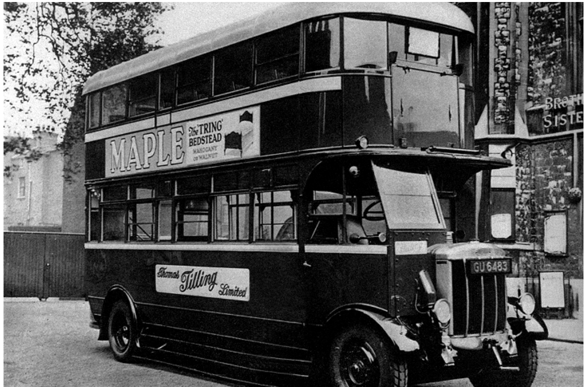
Tilling-Stevens' last passenger petrol electric offering emerged as the dropped frame TS17A, essentially a two axle version of the TS15A. Two 16 ft wheelbase double deck examples were operated experimentally in 1930 by Thomas Tilling in London. (LTHL collection).
