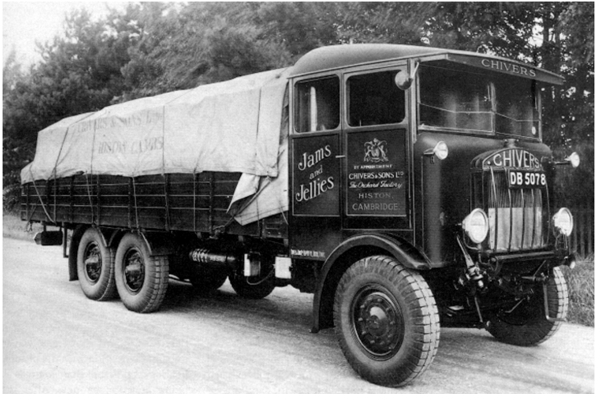
One of the Chivers conversions that could only have been undertaken in close co-operation with the Tilling-Stevens factory, and it is probable that the extensive reconstruction incorporated features adopted earlier in the six wheel TS15A design of 1928. (LTHL collection).
