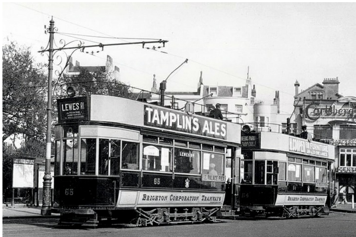
Cars 64 (behind) and 65 (front) were Brighton built cars that seated 52 and dated from 1928. They remained in service until the demise of the system in 1939. (LTHL collection).
