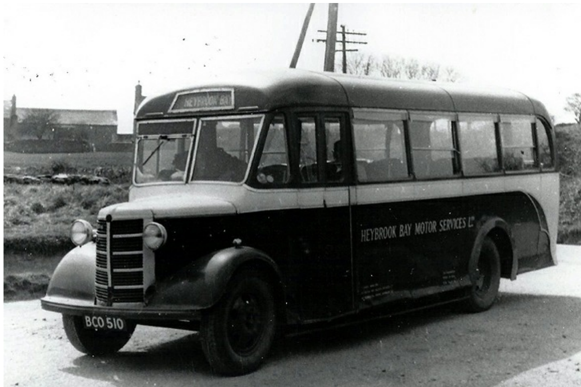
BC0510 was a 1938 Bedford WTB with Waveney? 24-seat bodywork, that was one of three vehicles acquired with the business of Star Motors in 1943. (LTHL collection via Roger Grimley).
