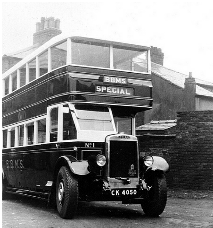
No. 1 (CK4050) was a 1928 Leyland TD1 acquired second-hand from Preston Corporation in 1938. It carried Leyland 51-seat lowbridge bodywork. (Prescott family collection).
